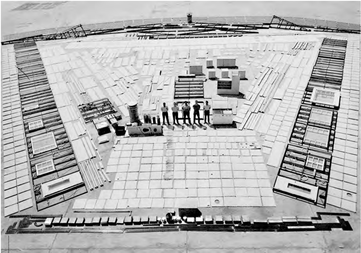
Figure 2. A Lustron house kit spread out on an airport runway to demonstrate the extensive contents of a Lustron House kit of parts. (ca 1950)
