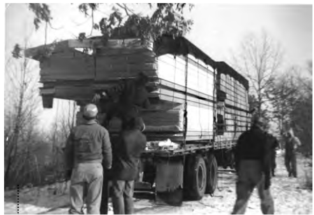
Figure 3. Techbuilt panels arriving by truck
