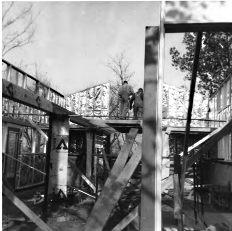
Figure 4. View of the erection of interior post and beam elements
