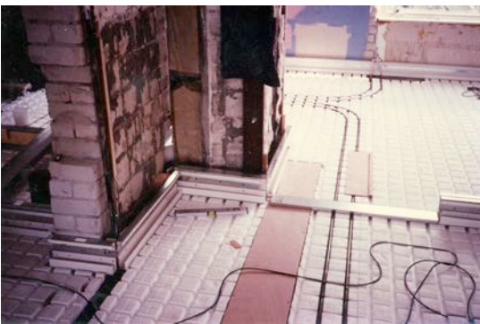
Matura lower system being installed
