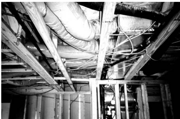
Fig.1 The entangled service systems in the floor cavity of a normal residential project, 1993.
