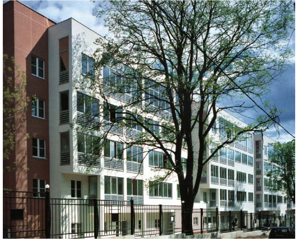
Catamaran House in Moscow, 2005 Reserve Architects / Vladimir Plotkin
