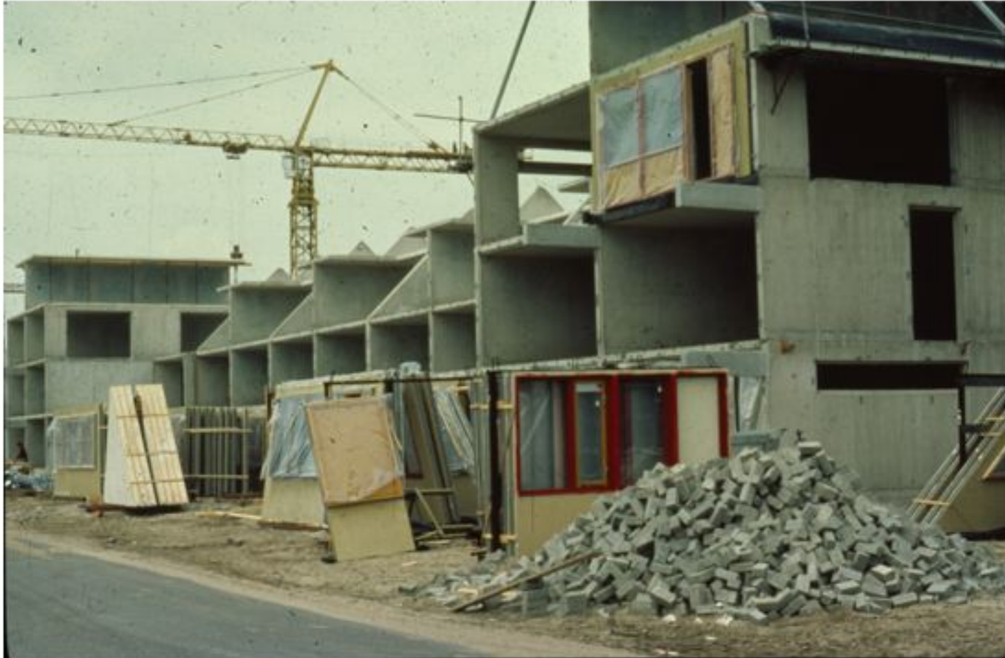
Tunnel form construction of the base building... and prefabricated façade panels
