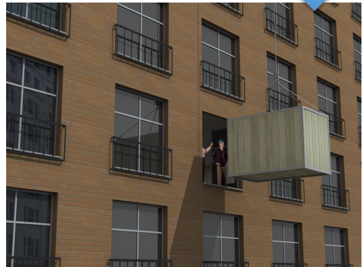
Container temporarily located
