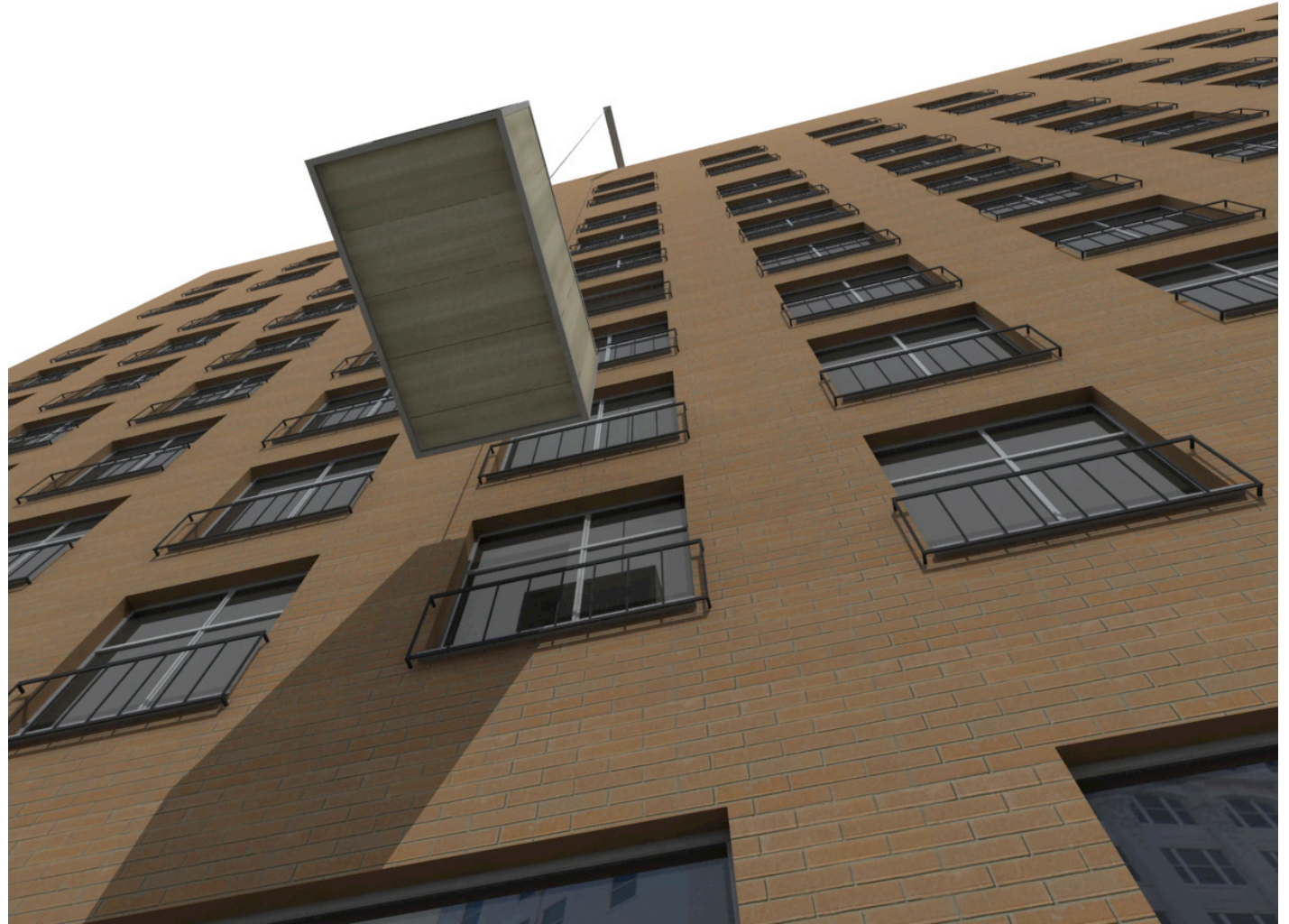
Lifting the container to the window for unloading.
