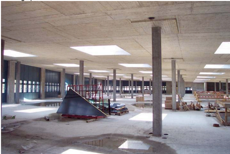
Figure 7: Interior view of the top floor of the empty Primary System, showing skylights, openings for light-wells to the floor below (on right of picture) and pre-cast columns with four sleeves at the base of each column for possible vertical drainage piping. Also visible is the inner layer of the double skin envelope showing operable wooden windows.
