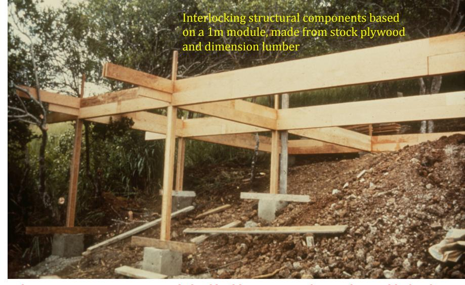
...houses in Puerto Rico, using a hybrid building system...designed to enable families to design their own houses. Elements were designed for any house, based on a dimensional module and a standard kit of parts...
