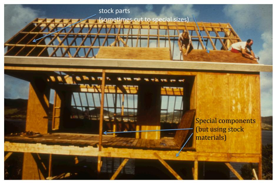
both stock parts and the special post-and beam components and wall panels...
