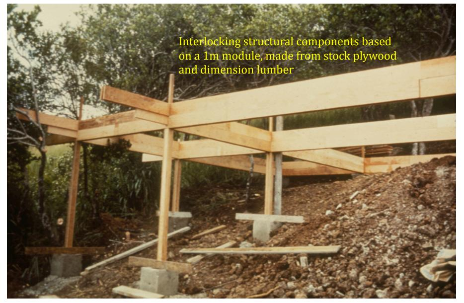
...houses in Puerto Rico, using a hybrid building system...designed to enable families to design their own houses. Elements were designed for any house, based on a dimensional module and a standard kit of parts...
