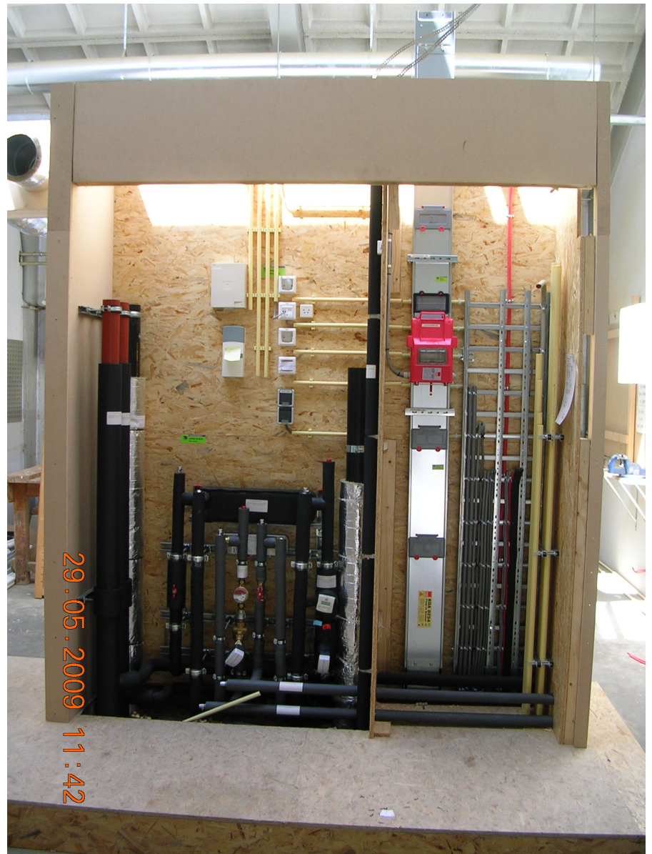
Examples of building utility cabinets
