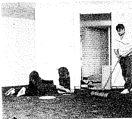
Figure 10. Installation crew at work.
