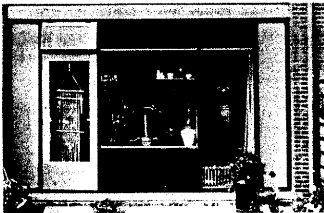
2.4 Two facades illustrating the variety achieved with a standard window frame which is identical throughout the project, and choice of infill by doors, windows, glass, or opaque panels.
