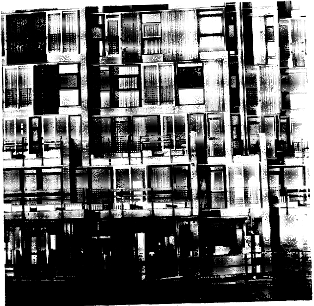
Figure 2. East elevation of "la Mémé"; arrangement of components reflects the arrangement of the rooms.
