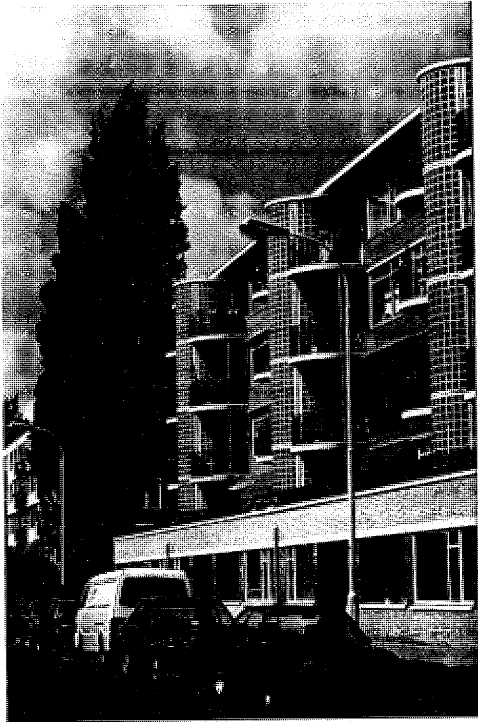
The Voorburg project showing the renovated base building, with new, enlarged balconies and stair, a new elevator at each stair hall, and new efficiency units facing the street on the ground. Architect: Henk Reijenga
