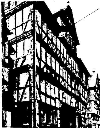
Half-timbered buildings could be built up, extended, taken down and moved; and then re-erected for another purpose on another site. Illustration from Matoko Suzuki's book Holzhauser in Europa.
