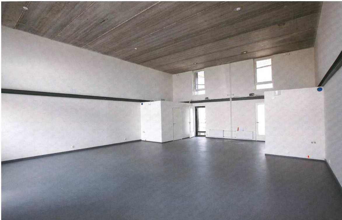
The empty shell space looking toward the front door and the two bathrooms installed as part of the base building. The piping hook-ups for kitchens are visible on the walls of the bathrooms – one or two kitchens can be installed, placed as selected by the inhabitants. Bathrooms on the upper level are also possible.
