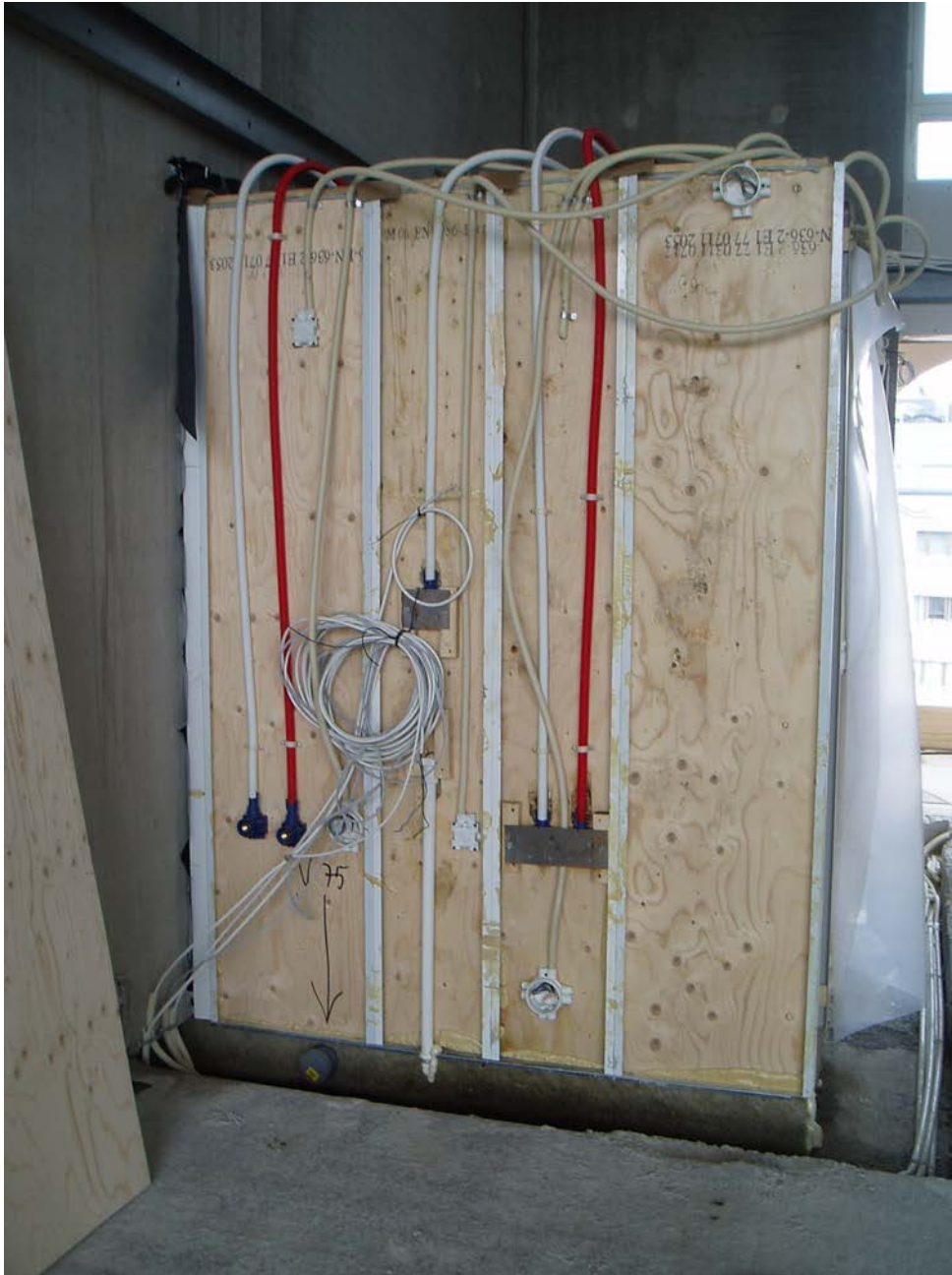
The bathroom unit in place
