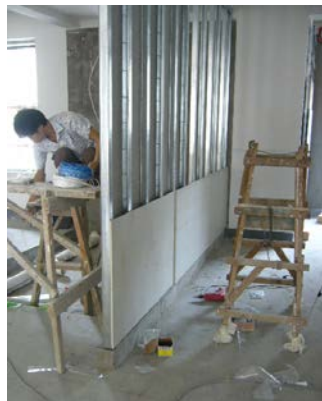
Metal stud/gypsum board interior partition
