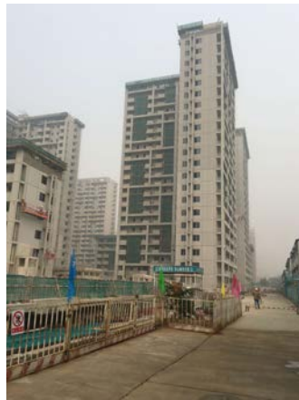
One of the apartment blocks using PREFAB infill
