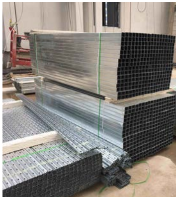
Metal studs made by PREFAB, bundled and labeled per building/floor/unit.
