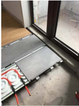
PREFAB's patented raised floor with floor heating
