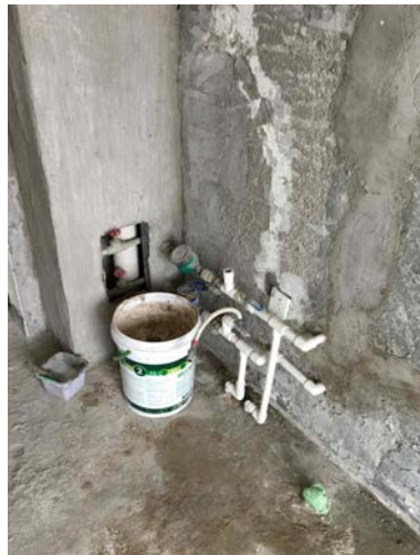
Drain from the WC + shower in the apartment above +new wiring and water lines
