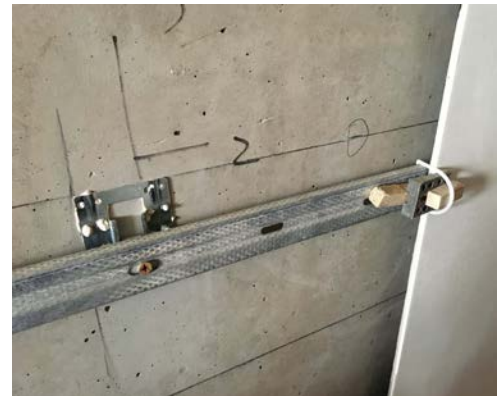
A patented method of attaching wall liners using adhesive (to reduce noise)
