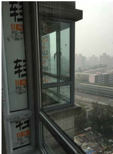
New window units having been installed
