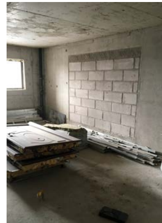
An empty unit receiving delivery of infill parts
