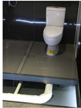
A display view of the raised floor
