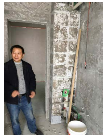
One of the workers beside the vertical pipe shaft
