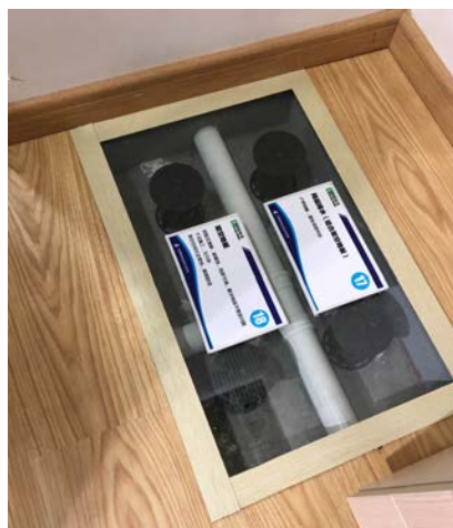
Another companies' raised floor solution
