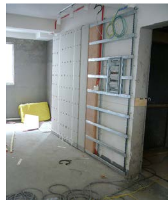
Special steel channels used as wall-liners
