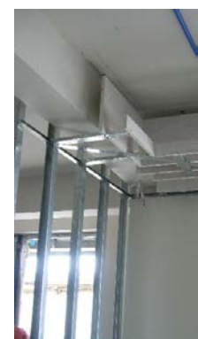
Metal stud work at the ceiling
