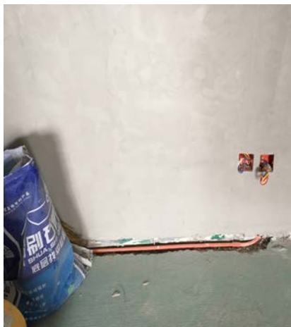
A new electrical conduit in a trench cut into the slab
