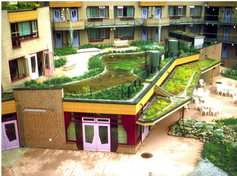
Figure API-5 View of the Restaurant Roof and the Yard
