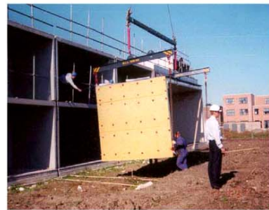
Installation of the facade module
