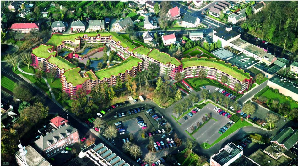
Figure API-1 Building in the Neighborhood
