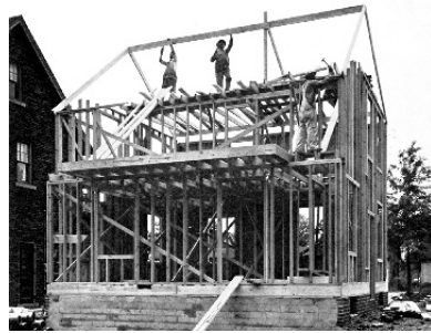
Fig.2 A balloon frame house in 1935. ( The Architectural Record , August 1935.)
