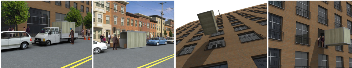
FIGURES 6-9: Delivery and unloading of contents into the unit to be fitted out.
