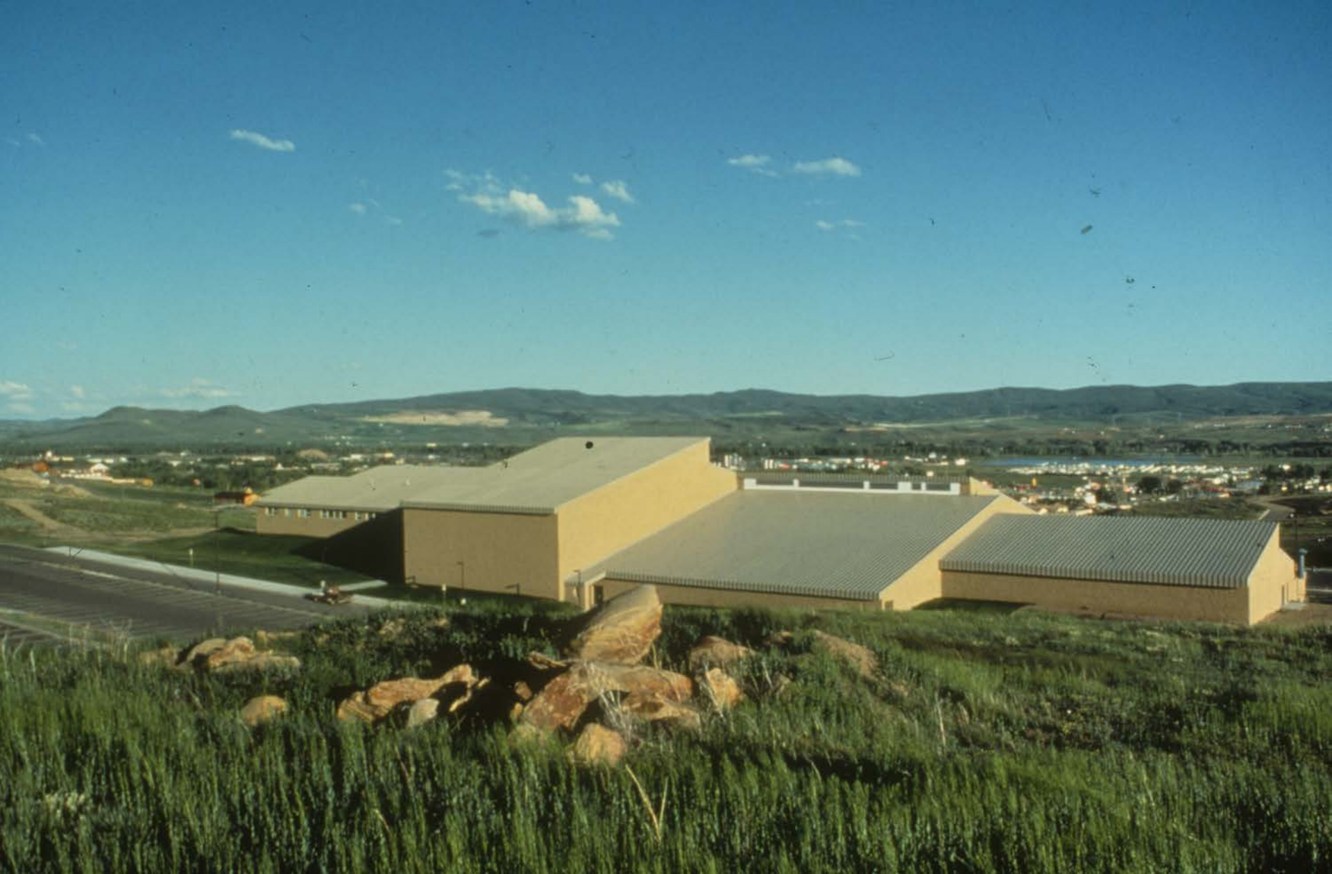
Moffat County, High School, Moffat, Colorado – 1980-82 (I was the project designer)
